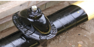
Fig. 5. Insulation of welding heads on the factory pre-insulated valve (no valve box) with surface operating rod
