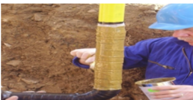
Fig. 6. Insulation of underground/surface transition fitting
