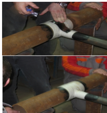
Fig. 3. Insulation on a tee (branch) with PE +BR strips (the two-strip system)
